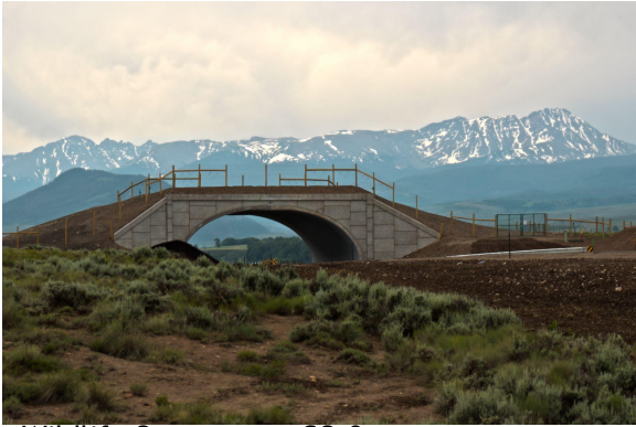
Wildlife Overpass on CO-9
