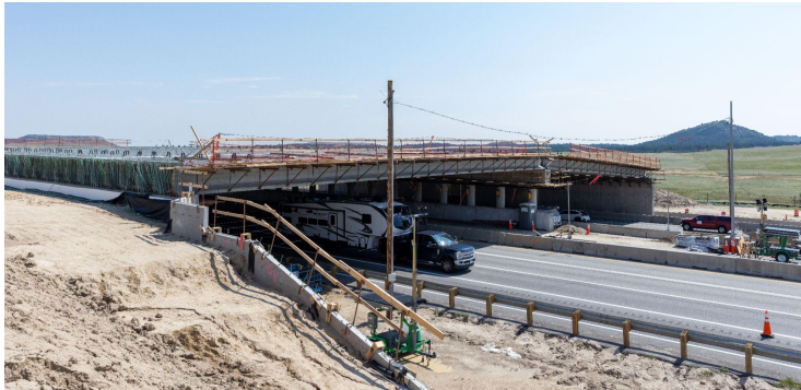
I-25 Greenland Wildlife Overpass under construction
