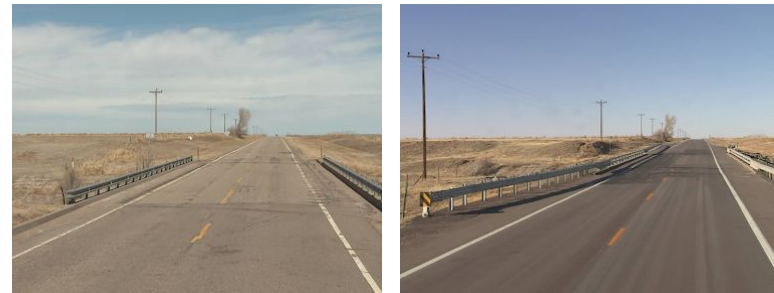
CO 59 South of Cope to I-70, Before and After Condition
