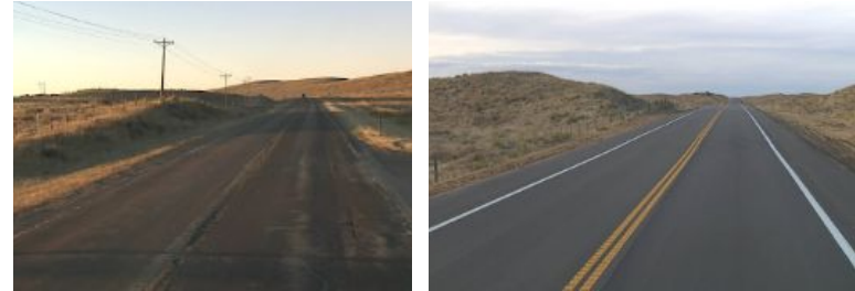
US 385 Phillips/Yuma, Before and After Condition
