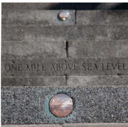
In 1969, engineering students from Colorado State University resurveyed the steps and determined that the mile-high step was actually the 18<sup>th</sup> step and a second marker was installed. A final attempt to precisely locate one mile above sea level was made using the new national vertical datum. Surveyors identified the 13<sup>th</sup> step as one mile above sea level. A third marker was installed and dedicated on September 29, 2003.
